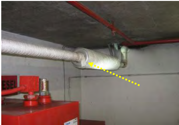
Photograph 15. Basement level P5: Fire Sprinkler Pump room - Woven SMF/glass wool band seal to exhaust pipe from diesel pump motor
