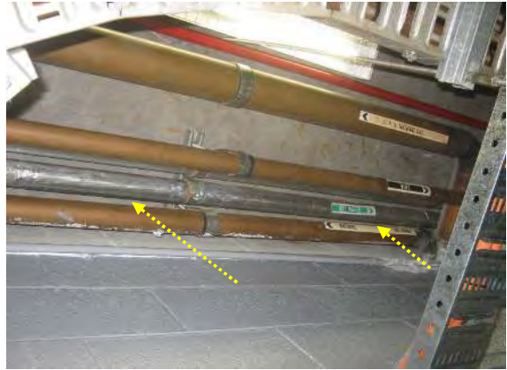
Photograph 16. Basement level P3: ST011 room (Cleaners); Hot Water unit ('Rheem'; 315L) - Internal cladding insulation (SMF based)
