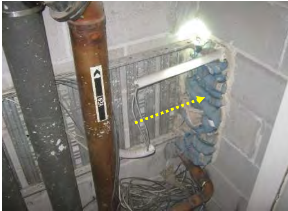
Photograph 15. Basement level P5: Fire Sprinkler Pump room - Woven SMF/glass wool band seal to exhaust pipe from diesel pump motor
